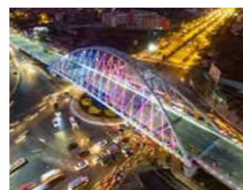
Haiphong (VN): A bridge for a safe traffic flow
